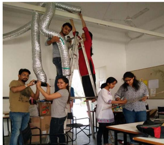
Figure 6 Installation of the HRV in class
