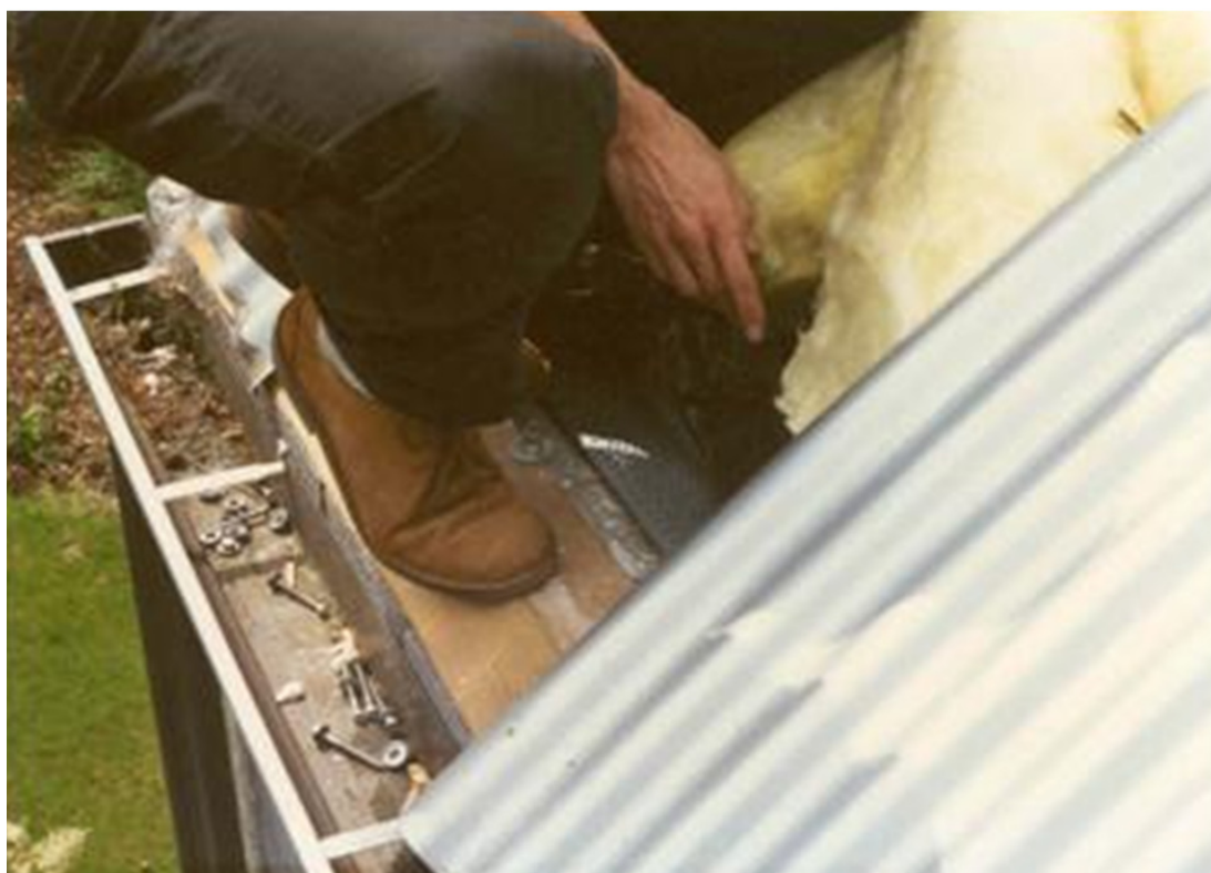
Figure 12: Opening the roof
