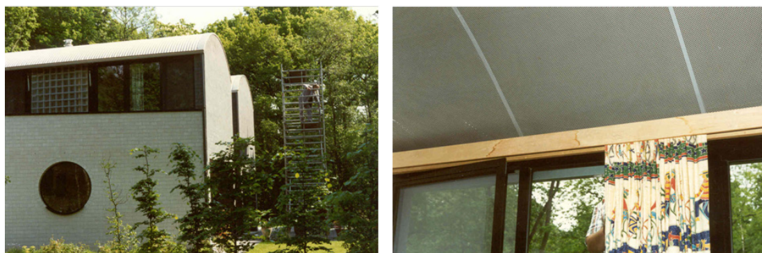
Figure 11: The house, ceilings consisting of perforated steel, traces of run-off on the pelmet board
