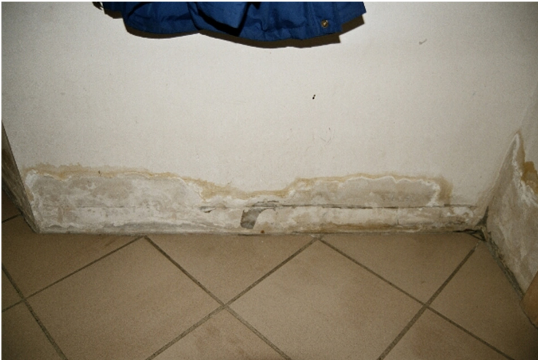
Figure 14: Rising damp in the inside walls
