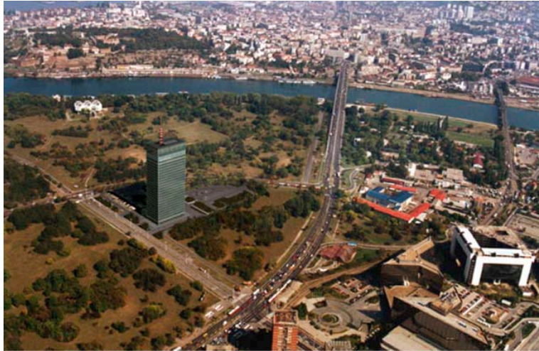
Fig 2 General view of the tower's site
