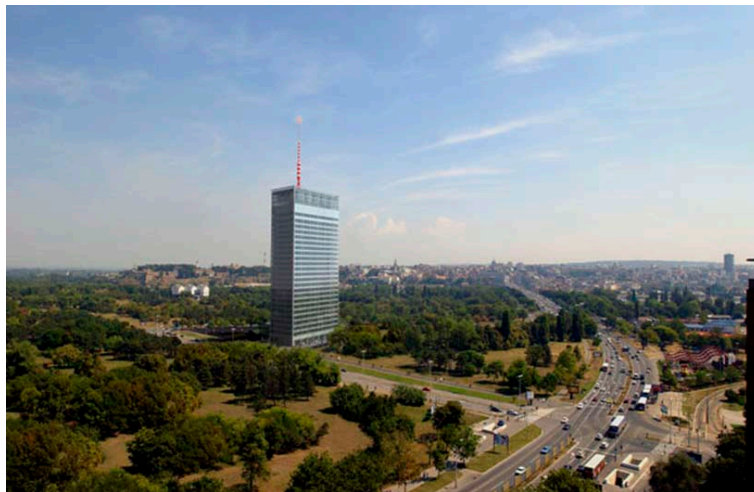
Fig 1 General view of the USCE Tower in Belgrade
