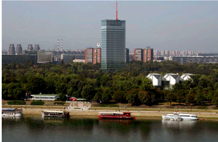
Fig 5 USCE Tower view from river
