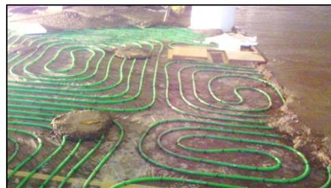
Figure 4- Radiant floor cooling system
