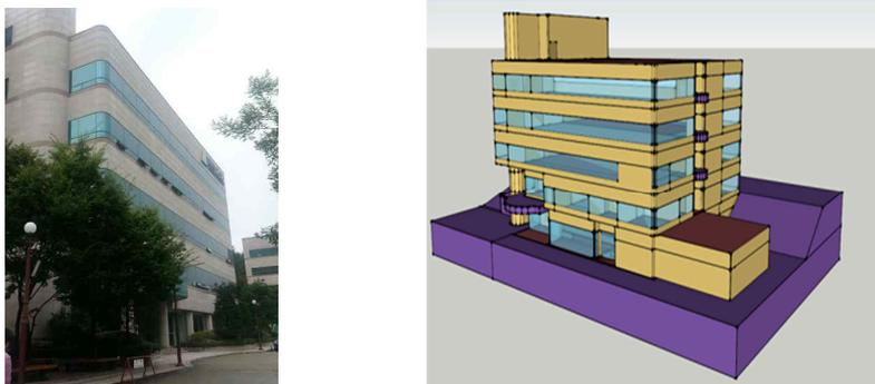
**Figure 1.** Target building (left) and EnergyPlus displayed in OpenStudio (right)
